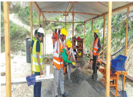
Construction Work in Progress at Durgamalinga.S.S
