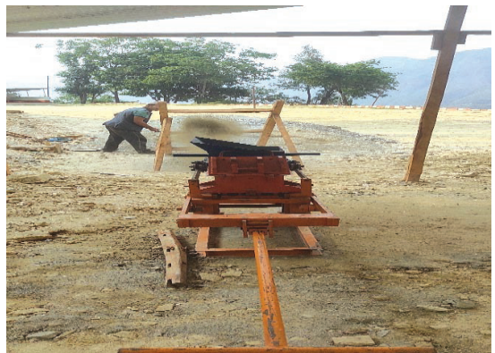
CSEB Brick Production Machine Set up at Construction Site
